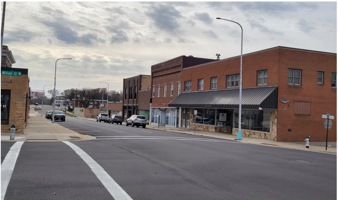
Top: View of the two primary facades on the corner Post Office building looking northeast circa 1940s. (ebay.com) (2.2.B.2) Bottom: View of typical street-facing primary facades in the district; the side street-facing facade on this corner building may be considered as secondary, 2023. (MacDonald & Mack Architects) (2.2.B)
