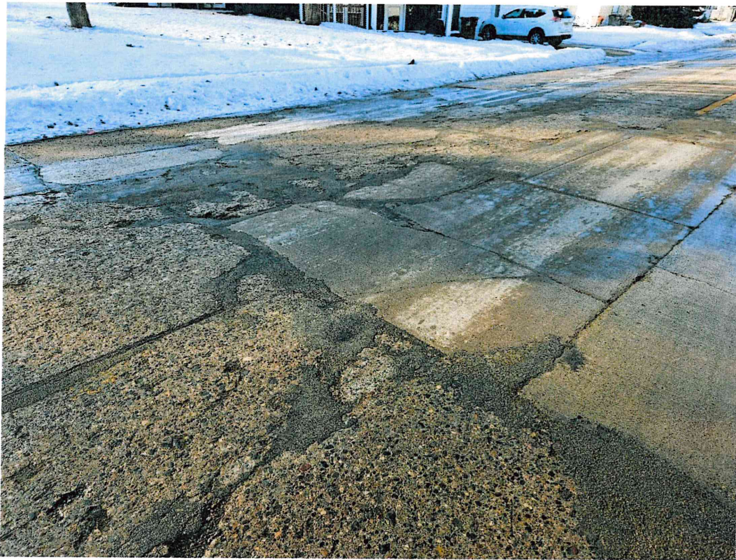
Figure 1 – Valley Avenue: Deteriorated concrete pavement
