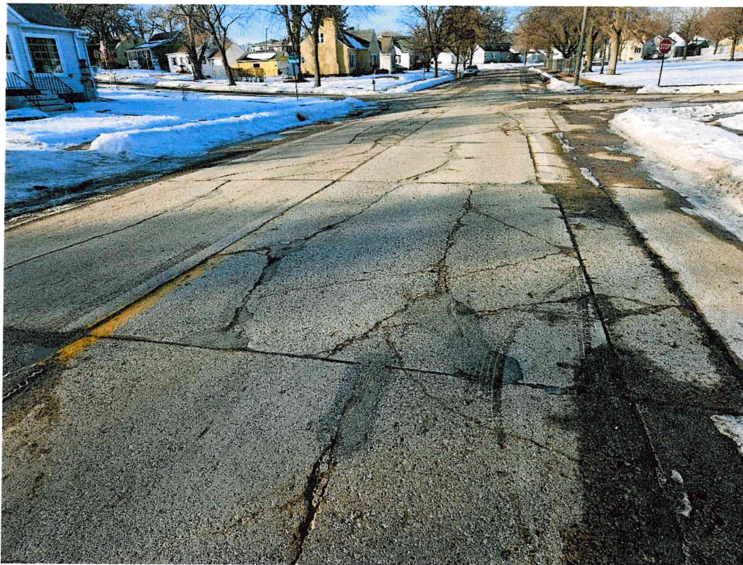
Figure 2 - Valley Ave: Deteriorated concrete pavement
