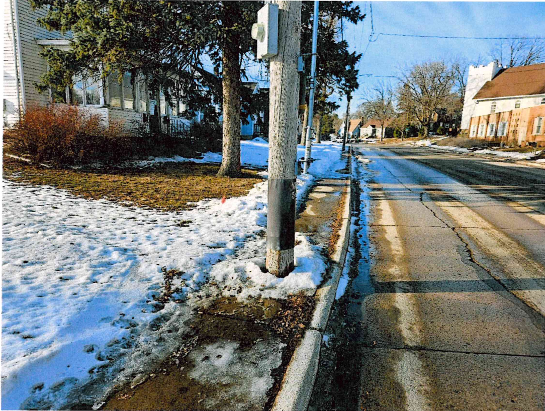
Figure 3 – Marshall Street: Obstructing utility poles to be relocated and affected trees removed
