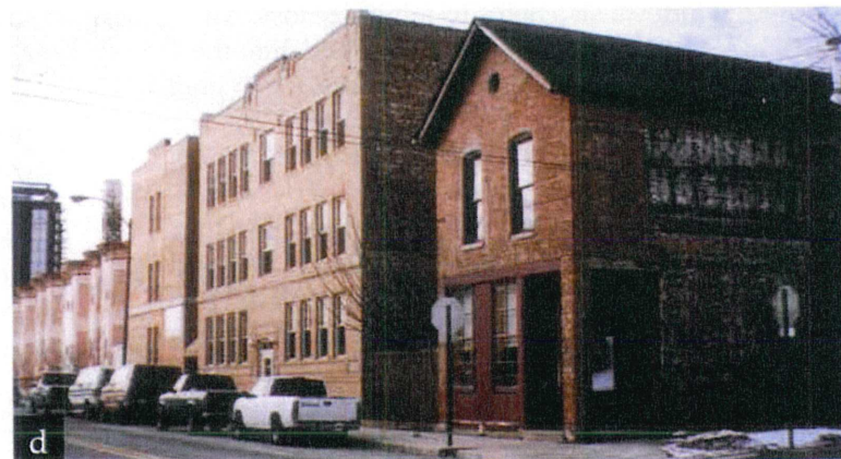
Figure 5. This addition (a) is constructed of matching brick and attached by a recessed connector (b) to the 1914 apartment building (c). The design is compatible and the addition is smaller and subordinate to the historic building (d).
